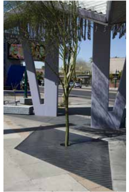
Mesa Transit Station Tree Grating
