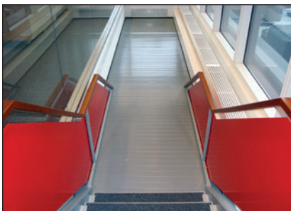
The handrail riser configuration of a non-egress stair easily hosts the 2-hour shutter without compromise to the design.
