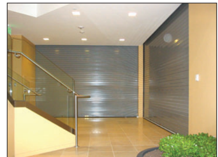
Openings in rated walls requiring temperature rise ratings are no longer limited to standard swing door dimensions when protected by the Model FSFD-TR, meaning greater design flexibility.
