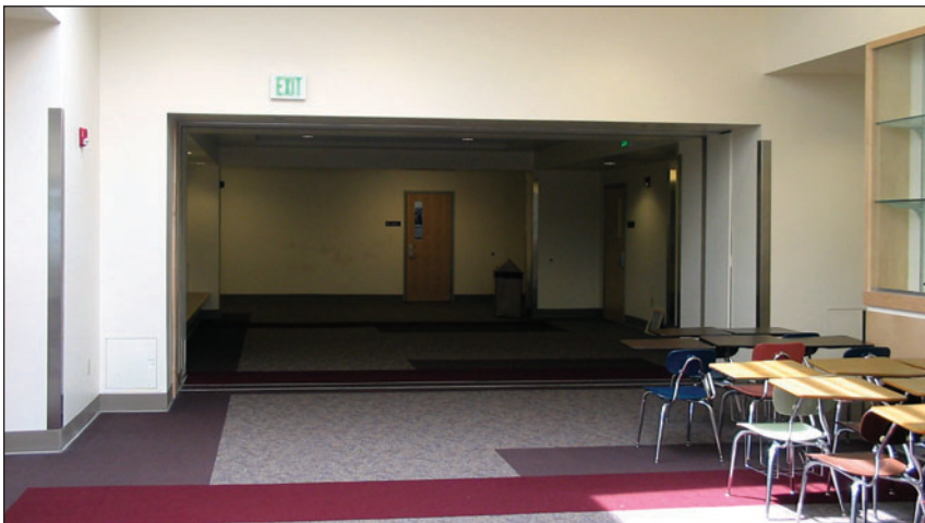
When the Safescape® S9500 fire door assembly is in the activated or fully closed position, egress is still possible through complying egress doors located at the leading edge.
