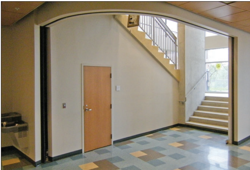
The Safescape® S9000 fire door retracts into a side pocket and is virtually undetectable when in the stored, fire-ready position.
